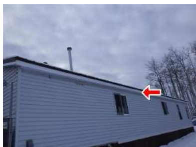
1.3 North Side Of Building
